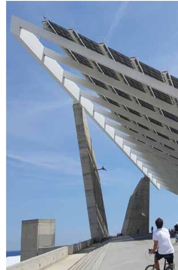
Roof by José Antonio Martínez Lapeña & Elías Torres Architects
