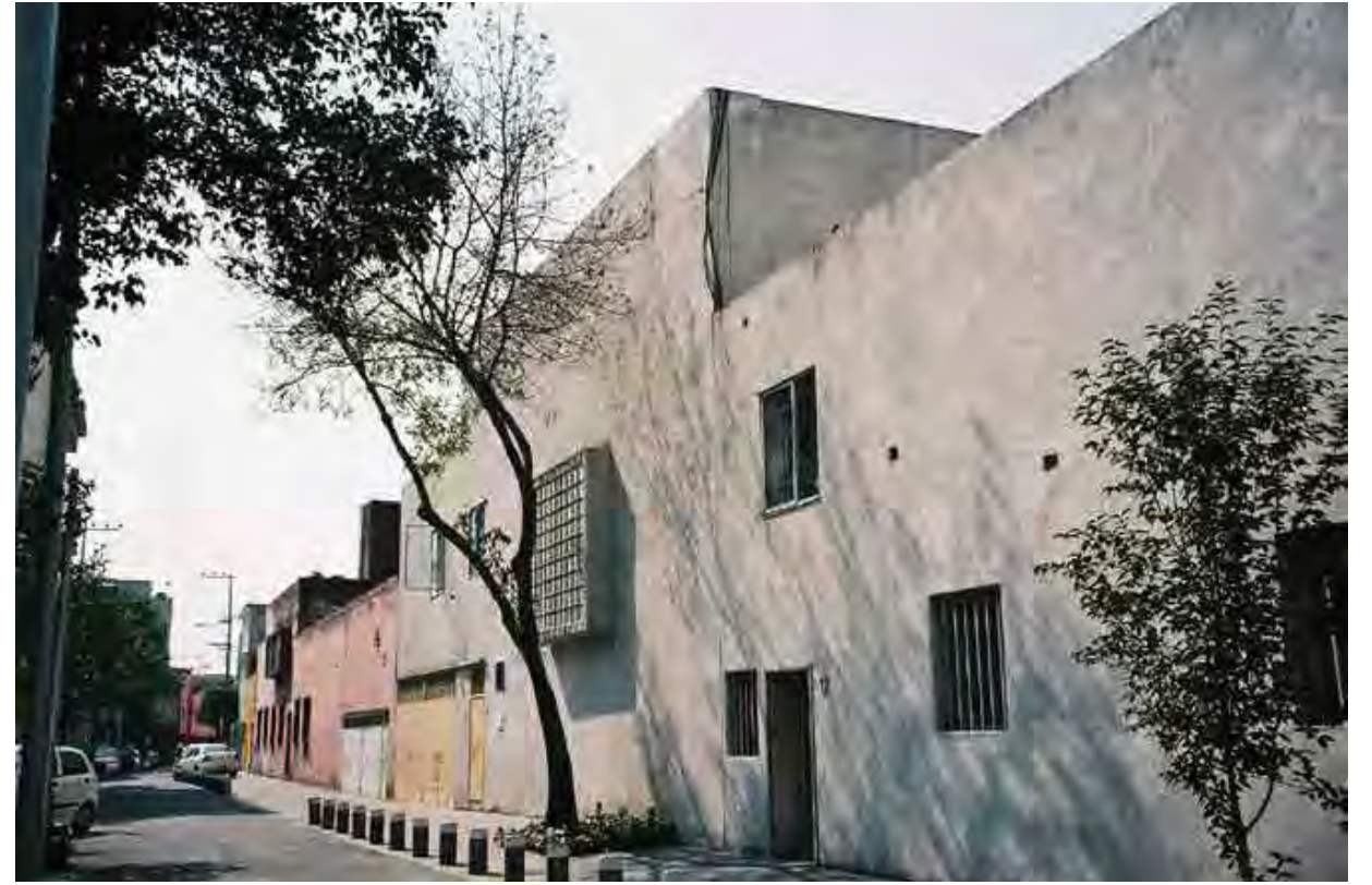
Barragan House & Studio, 1947-48, Mexico City.
