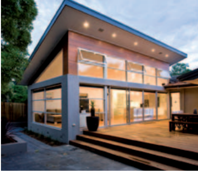
CREELMAN HOUSE TT ARCHITECTURE PHOTOGRAPHER: RED ZEBRA PHOTOGRAPHY
