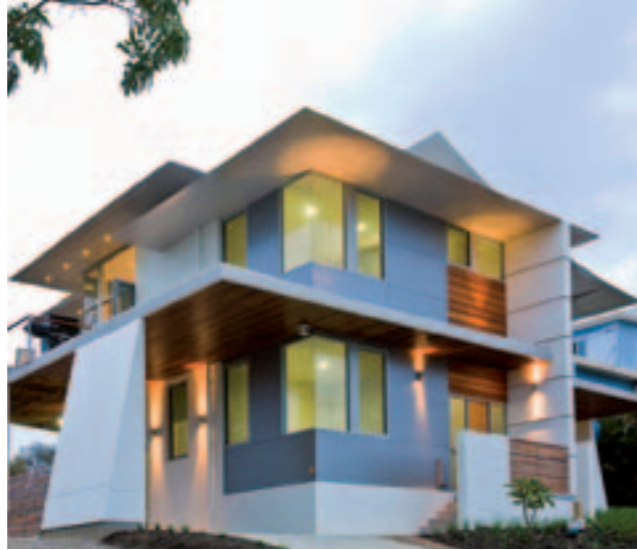
MALUA BAY HOUSE TT ARCHITECTURE
