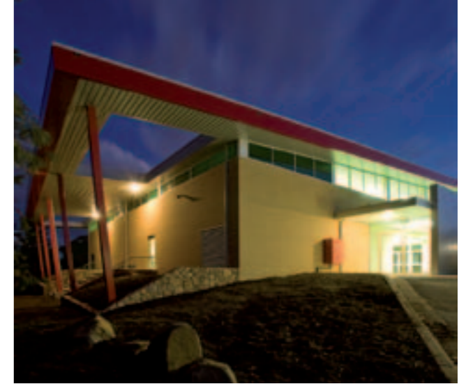
REFURBISHMENT – SACRED HEART PRIMARY SCHOOL, PEARCE AMC PROJECTS
