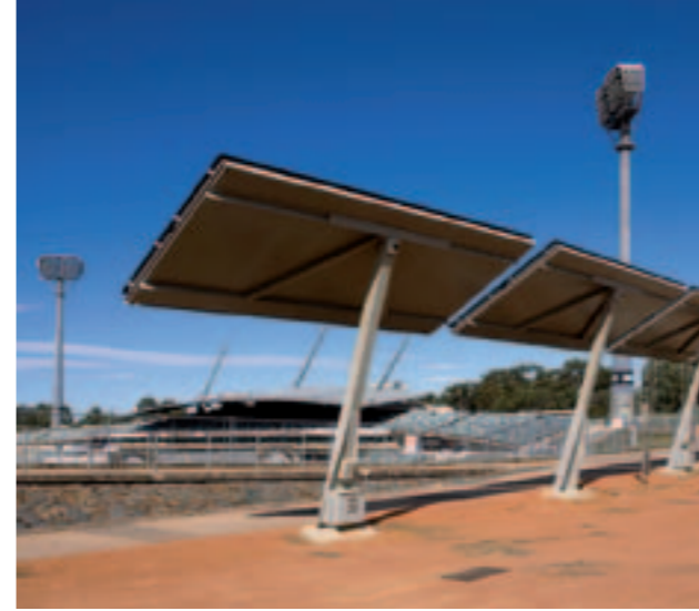
CANBERRA STADIUM SOLAR PANELS COX ARCHITECTURE
