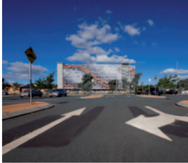
CANBERRA HOSPITAL CARPARK COLIN STEWART ARCHITECTS
