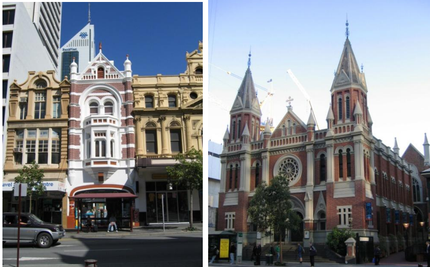
Trigg's Chambers, Barrack Street - the ground floor façade was altered, changing two round arches to form a single flatter arch, in 1979; Trinity Church, St George's Terrace (both John Taylor 2007)
