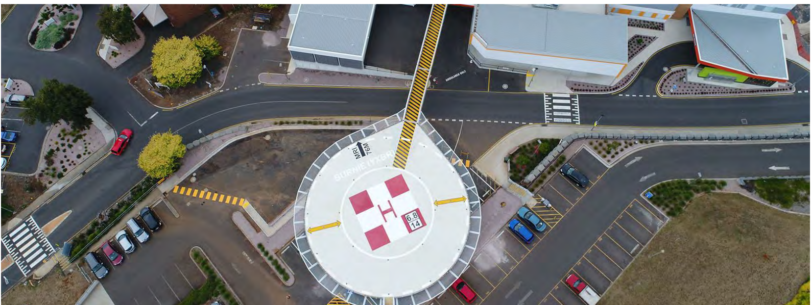
2017 Toyota National Civil/Infrastructure Award – under $25 million, AJR Construct, North West Regional Hospital Helipad, Tasmania
