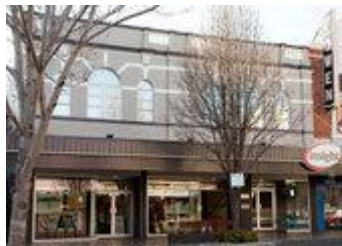
Insight Accountants by Aspect Architects and Project Managers. Image by Kingfisher Creative.
