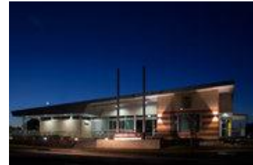
New Shire Offices Flinders Shire Council Hughenden by Tippet Schrock Architects. Image by Marguerite Leahy.
