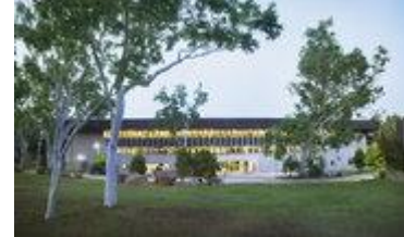
JCU Eddie Koiki Mabo Library Townsville by Brewster Hjorth Architects. Image by Rob Parsons.
