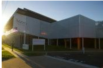
Mater Hyde Park Consulting Suites by Stephen de Jersey Architect. Image by Stephen de Jersey Architect.
