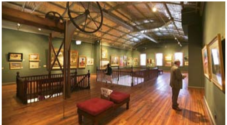
82 : The original curved roof has been lined, while still exposing the significant 1889 light metal truss.
